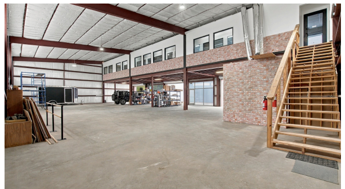
Stair access from the warehouse floor to the second-level offices.
